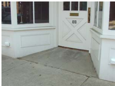
The slope of the pavement at this entrance eliminates a step.
