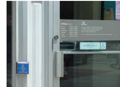
This entrance has an automatic door opener and is appropriately marked with the international symbol.
