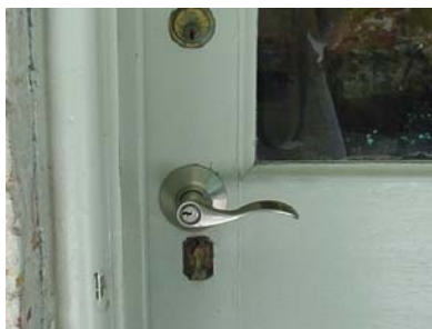
The hardware on this door has been converted to a lever that can be opened more easily.
